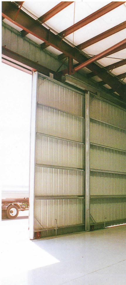
Standard Coporate Door & Wheel System. Shown is optional Galvanized Stiles & Girts.
