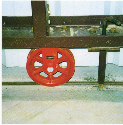
Standard Coporate Hangar wheels are 9" Shoulder Groove with grease fittings on 12" ASCE Railroad Rail.
