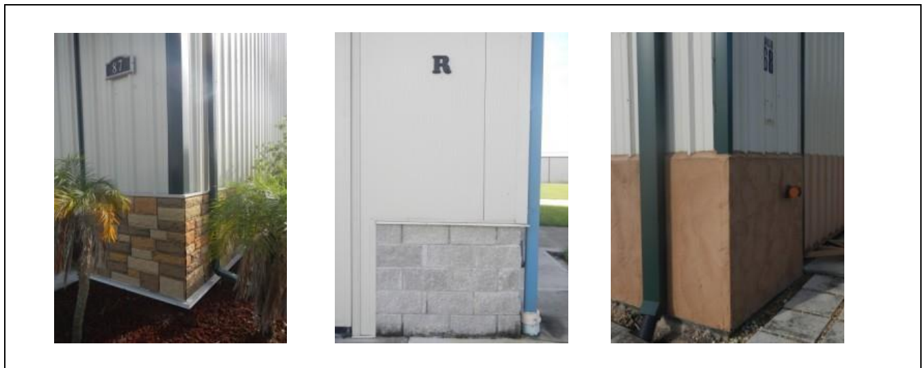
Hangar Outside Skirt - Typical Designs
